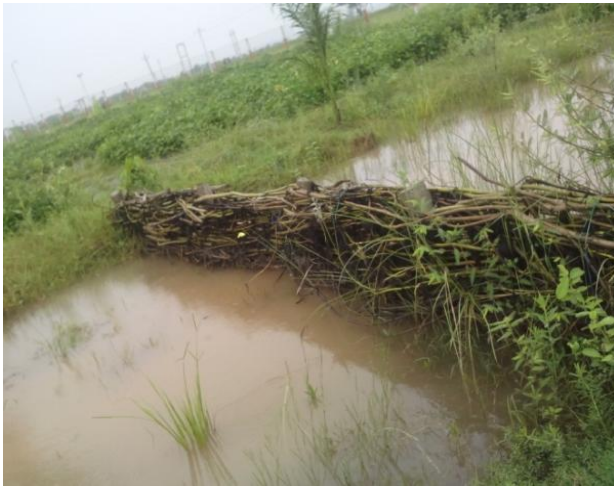
Fig 1: Single row brush wood dam
