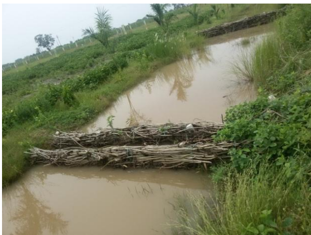
Fig 2: Double brush wood dam
